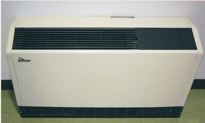
One of two ClimateMaster Tranquility® Console (TRC) Series units installed in ASHRAE headquarters.
