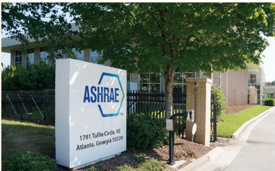
The exterior of ASHRAE headquarters
